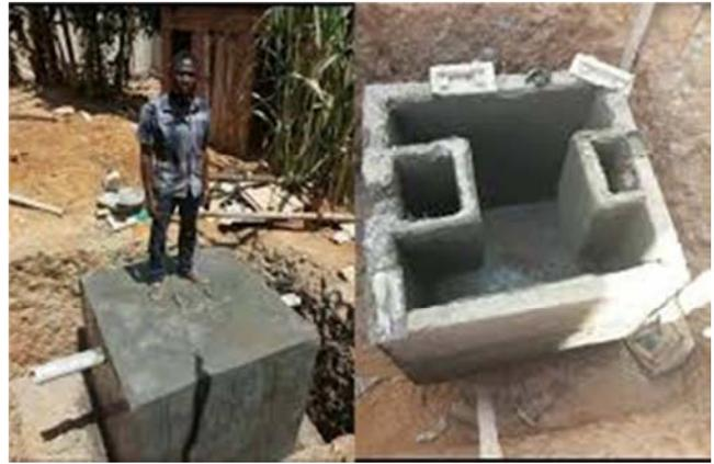
Figure 3. Construction of the biodigester (septic tank) system.
